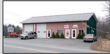
Bethel Commercial! $484,900 Fabulous business opportunity! 2 garage-bays, 3 units; Currently rented. 1± acre, high visibility on State RT-17B. Close to NEW "Bethel Woods" Performing Arts & Cultural Center & the "Racino" in Monticello (Proposed Casino Site). #19778
