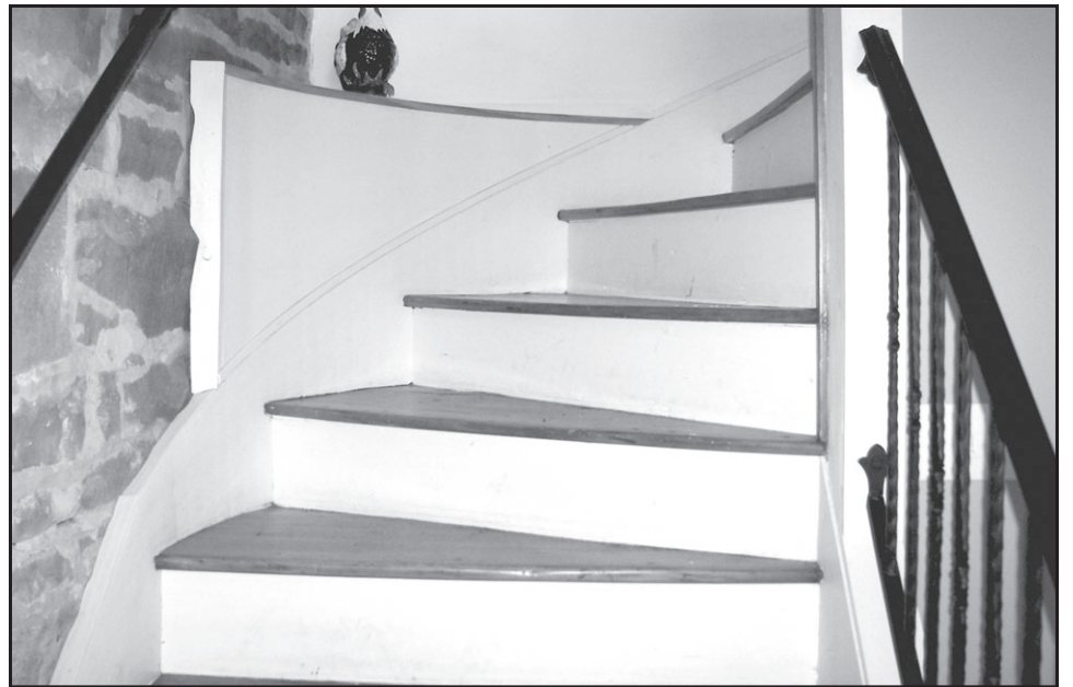
The original spiral staircase was salvaged and reinstalled during the remodeling.
